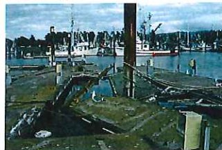
Damage to docks in harbor
